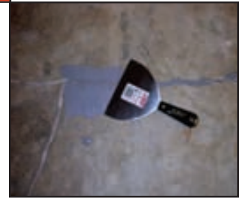
Fill Crack with VP Crack Weld
