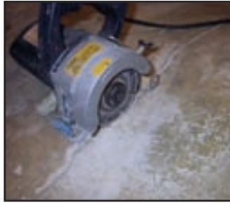
Open up crack with a crack chaser
