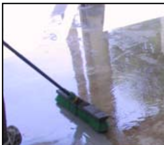
Use a Broom to Scrub Surface
