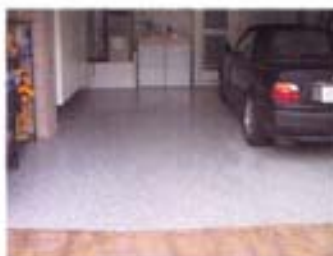
A Coating Systems Installation
