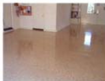
A Concrete Creations Installation
