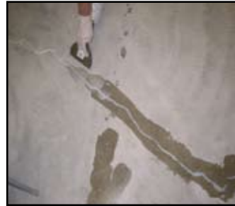
Trowel Epothane Into Crack
