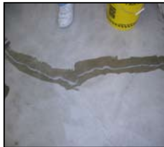
Crack Filled Flush With Epothane
