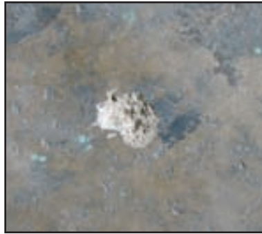
Spalled Concrete
