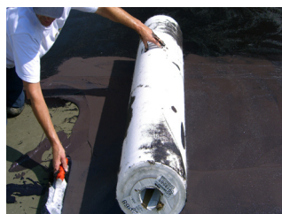
Trowel 1075 Membrane into 1075 Fabric
